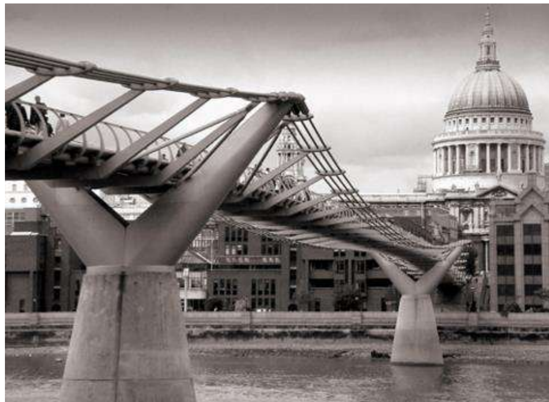
Millenium Bridge (2000), London, UK
