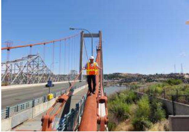
Maintenance Cables (New Carquinez)
