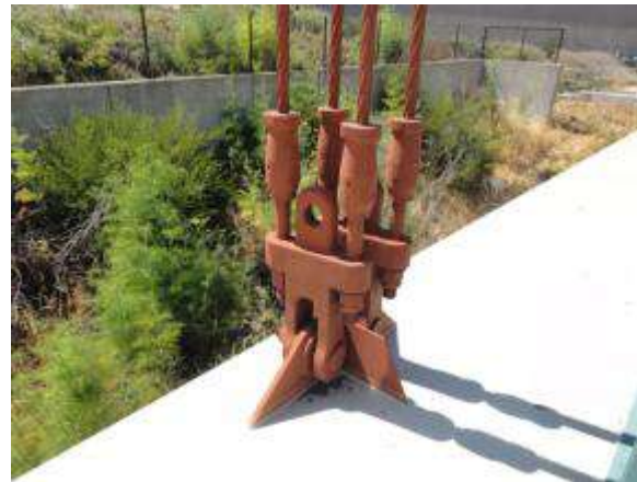
Hanger (New Carquinez)
