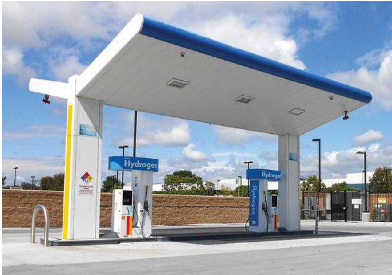
Gaseous hydrogen fuelling station, USA
