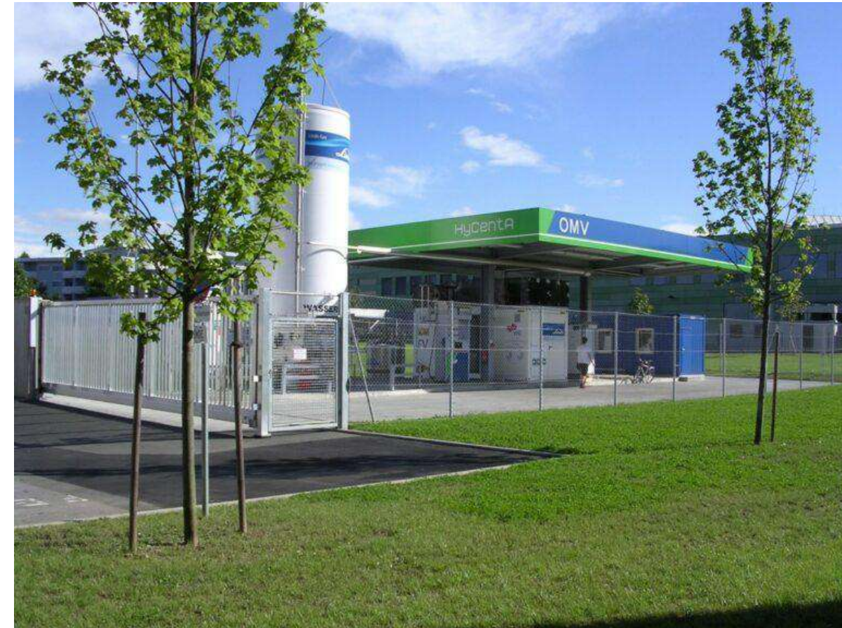
Gaseous hydrogen fuelling station, Graz, Austria
